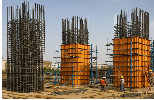
FIGURE I. 21. STRUCTURAL ELEMENTS WITH CLOSELY SPACED REBAR
