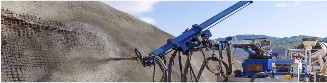
FIGURE I. 23. SHOTCRETE APPLICATIONS
