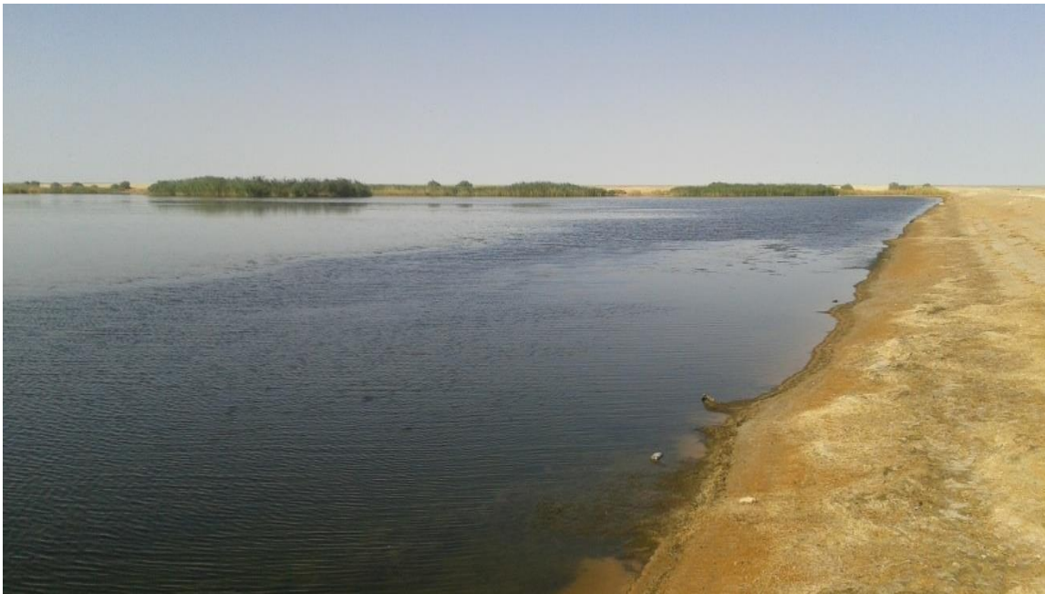
Figure 3.5: Treated Water Discharge Lake
