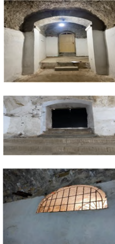
Figure. 9 Damaged carpentry elements.
