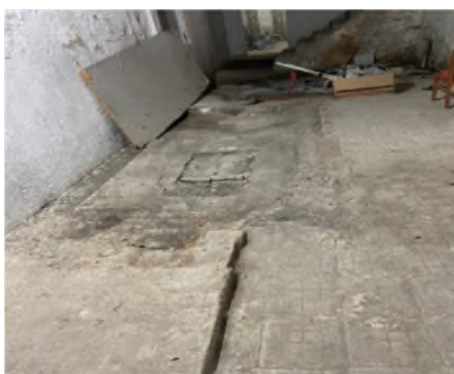
Figure. 8 Condition of the interior finishes.
