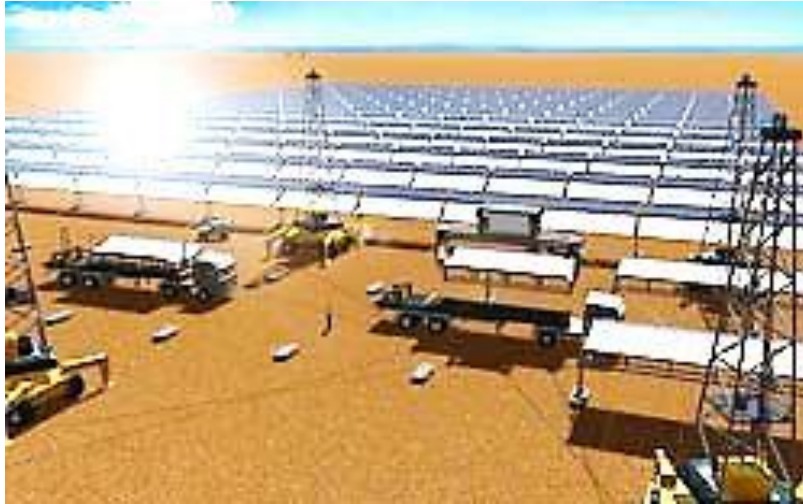
Figure I. 14. Vision of assembly of parabolic reflector panels with a mobile large-scale cable-driven parallel robot.
