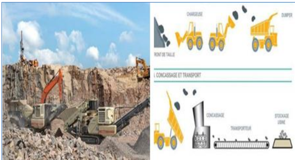
Figure I-5: Extraction et concassage
