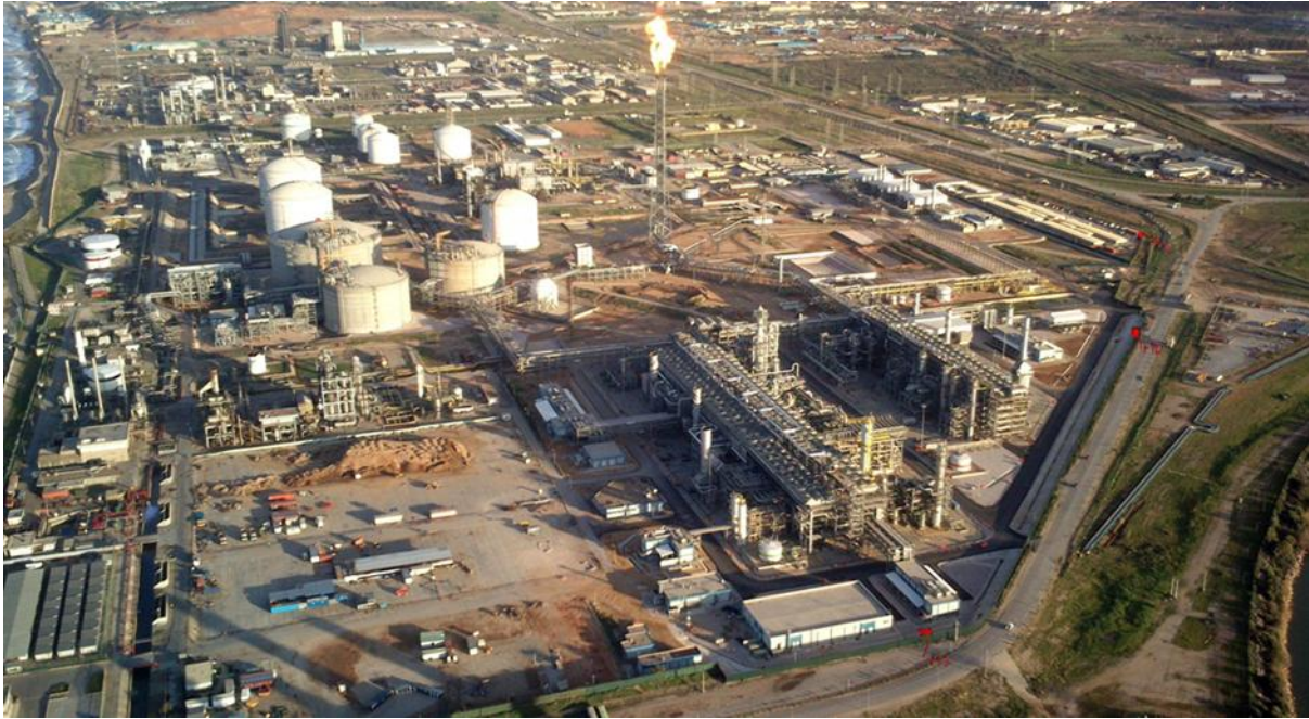
Figure II.1: The GL1K SKIKDA natural gas liquefaction complex
