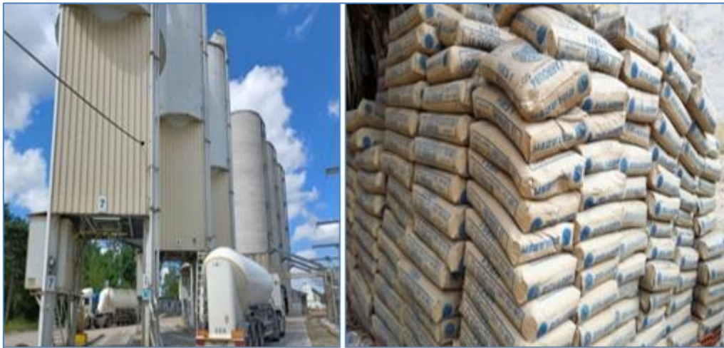
Figure I-6: Stockage du ciment
