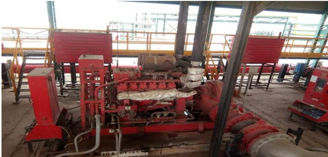
Figure III.10: Pompes diesel.
