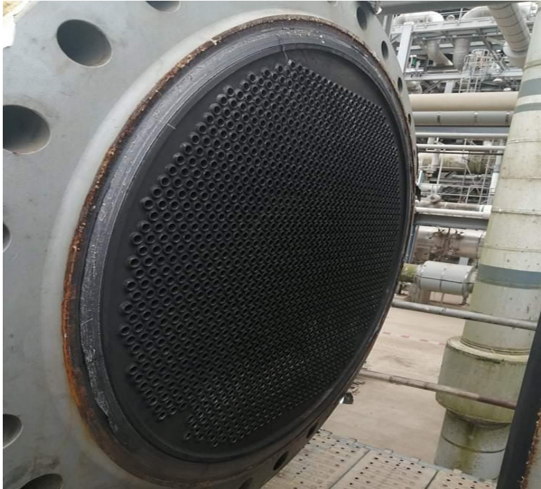
Figure (III.4): Tube/shell heat exchanger from Refinery 2 Sonatrach Skikda RA 2 K
