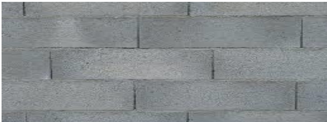
Figure I.3 : Support en parpaing.
