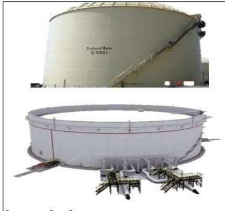
Figure II.4: Bacs de stockage cylindriques verticaux
