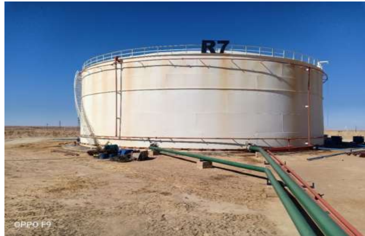
Figure I.23 Bac de stockage.
