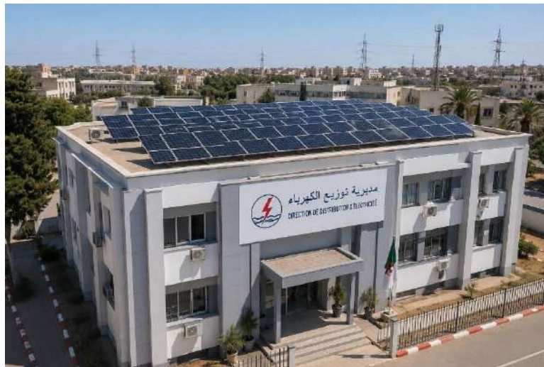
Fig.III.2. AI-Generated View of the Studied PV Installation.
