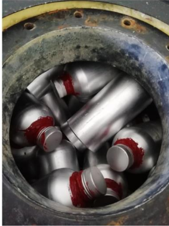
Figure I. 15 : The top view of the tank incorporates macro-encapsulated PCM [124].
