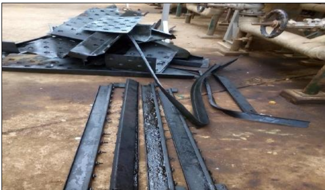
Figure III.10: C1 supports after a high vapor flow rate.
