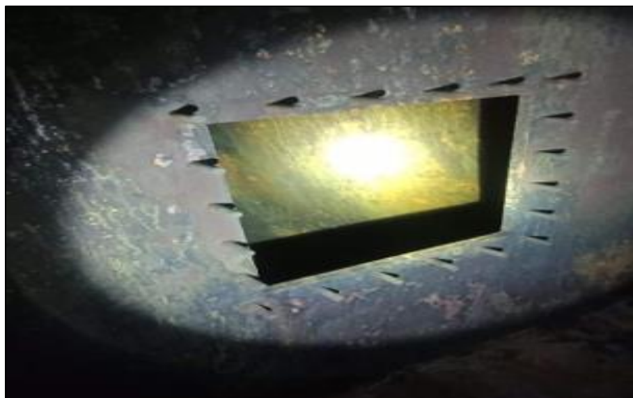
Figure III.12: Bottom Manway of the column C1.
