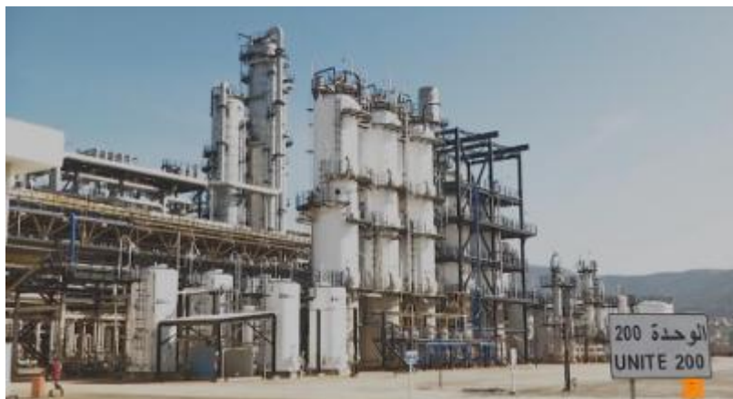
Figure I.3- Kerosen treatment unit (Unit 200)
