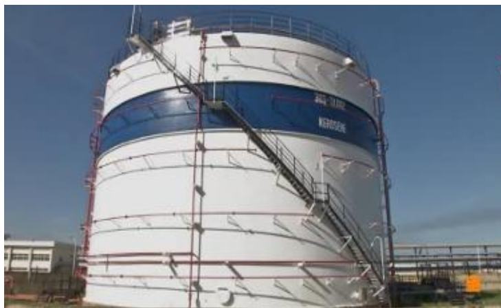
Figure I.4 -Kerosene Storage Tank
