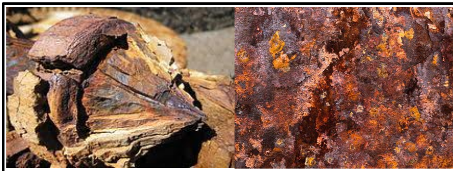
Figure I.3. La corrosion uniforme.
