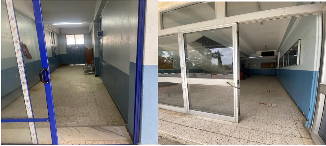
Figure :35 : Laboratoire de structures
