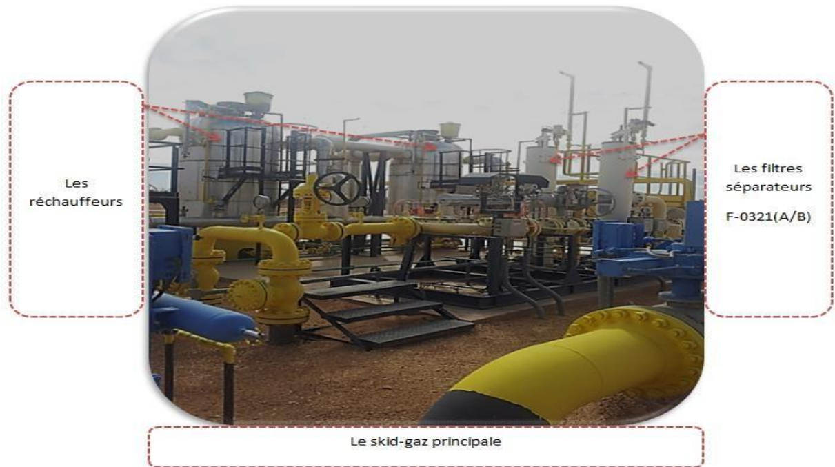
Figure I.9 : Skid gaz [8].
