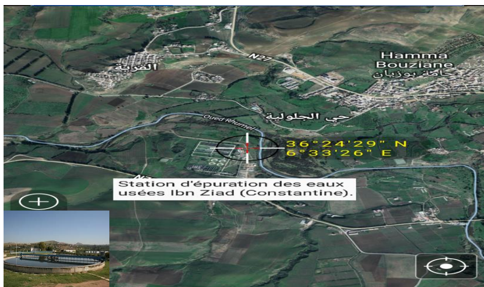
Figure III.4: Station d'épuration des eaux usées Ibn Zied.
