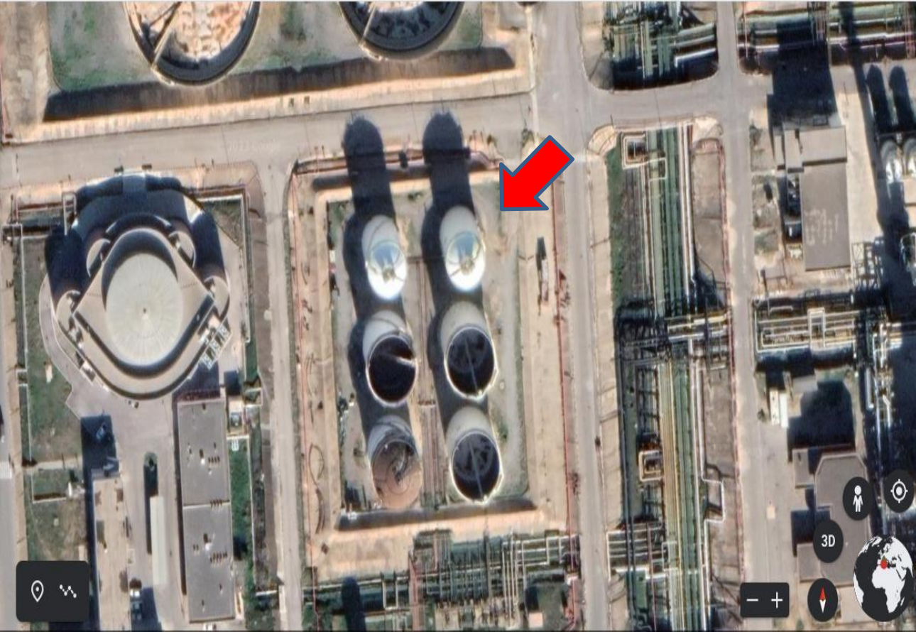
Figure IV.1: le bac de stockage S19 (google earth).
