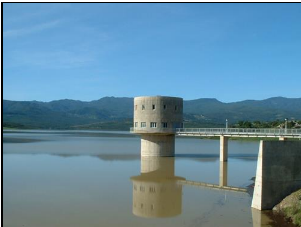
Figure 35 : Barrage Beni -Zid. [35]
