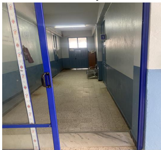
Figure :35 : Laboratoire de structures
