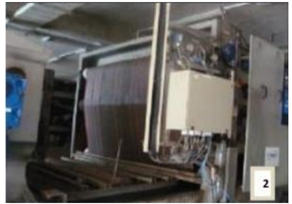
Figure 1.14: Drip Table (1) and Belt Filter (2) (Sidi Merouane Wastewater Treatment Plant, 2019)
