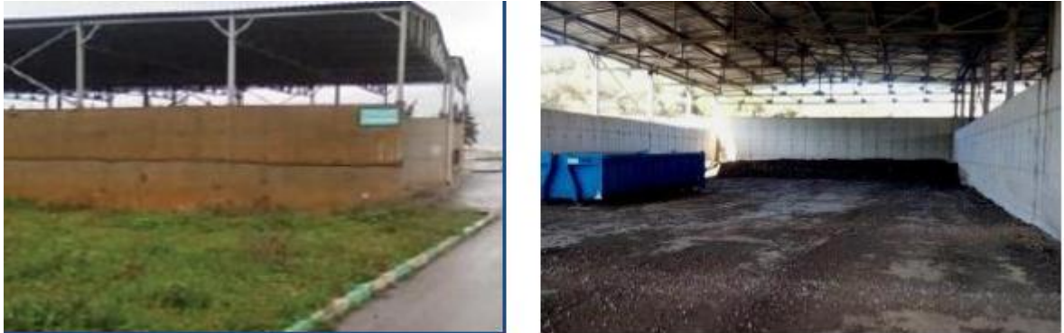
Figure 1.16: Storage Areas (Sidi Merouane Wastewater Treatment Plant, 2019)
