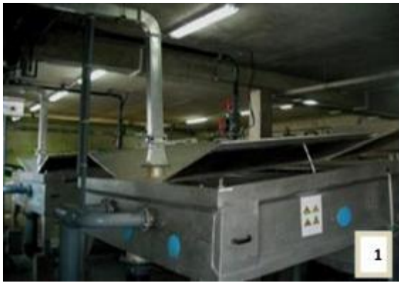
Figure 1.14: Drip Table (1) and Belt Filter (2) (Sidi Merouane Wastewater Treatment Plant, 2019)
