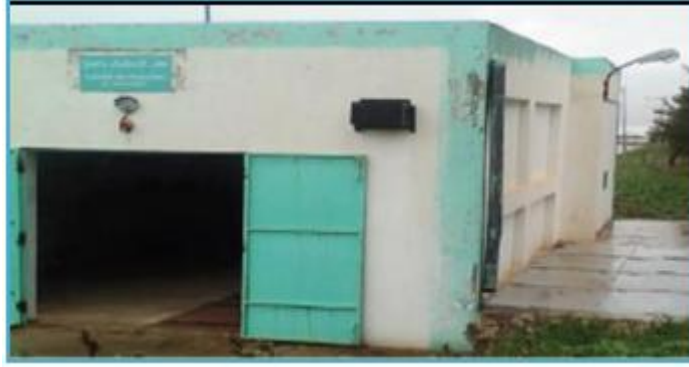
Figure 1.3: Reception and Pumping Station (Sidi Merouane Wastewater Treatment Plant, 2019)
