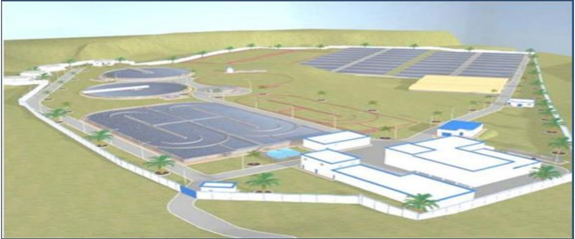
Figure 1.2: Overview of the Sidi Merouane Wastewater Treatment Plant (Sidi Merouane Wastewater Treatment Plant, 2019)
