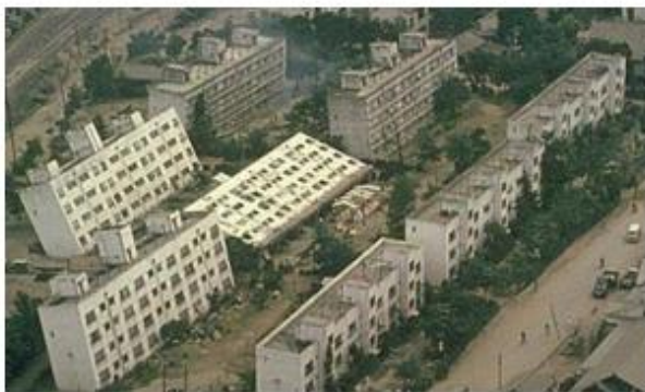
a) Building toppling Niigata 1964
