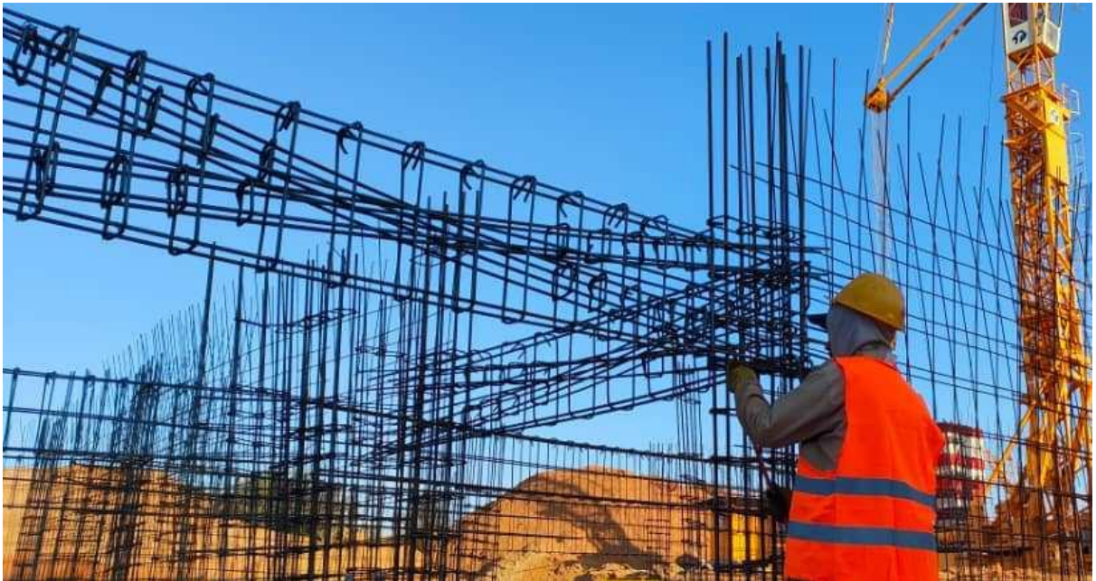
Figure I-3 ferrailage linteau voile
