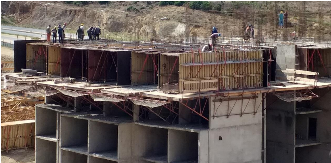
Figure I-1 Ferrailage dalle plane
