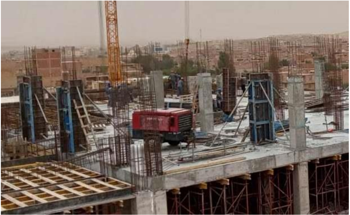
Figure I-4 Coffrage poteaux.
