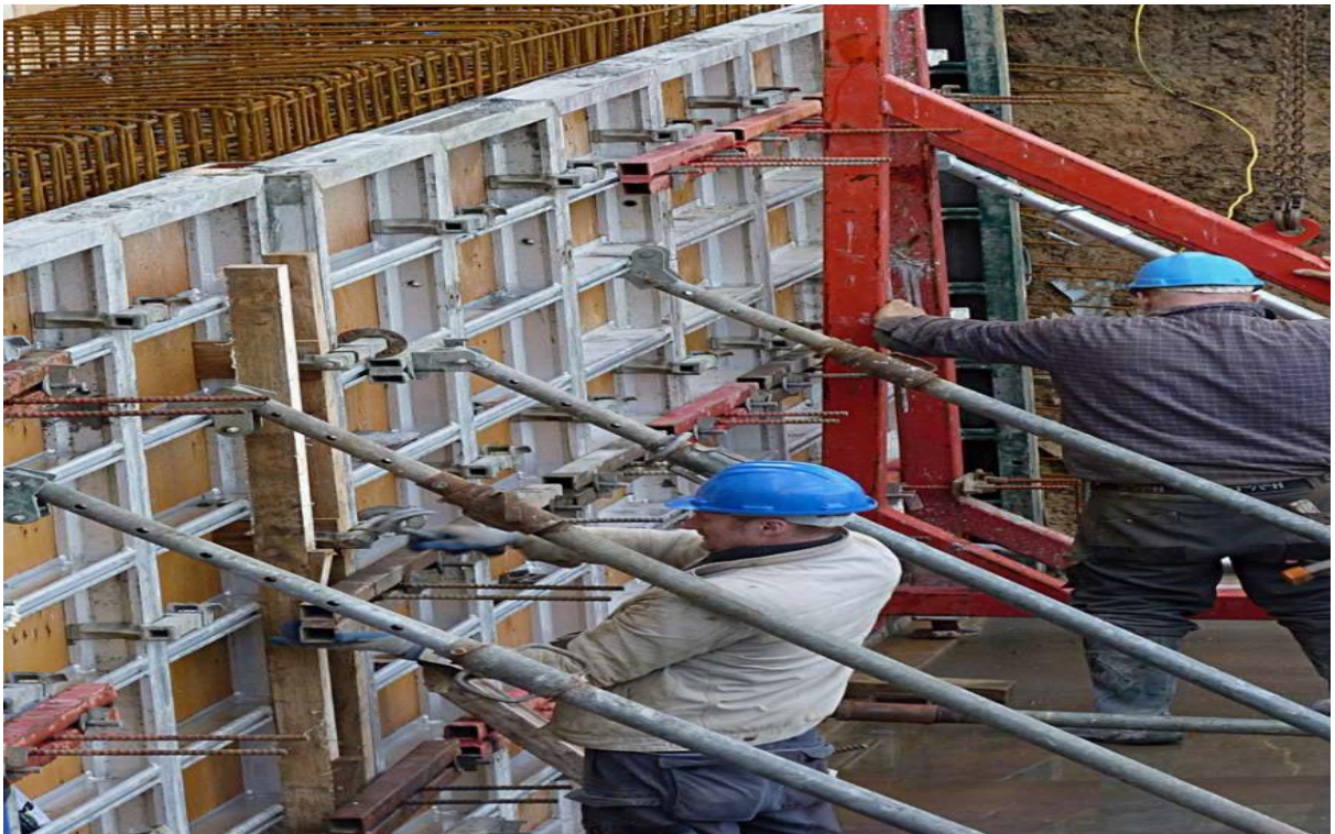
Figure I-5 Coffrage voile
