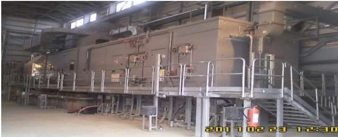
Figure II.16: Booster and lift Gas compressor.
