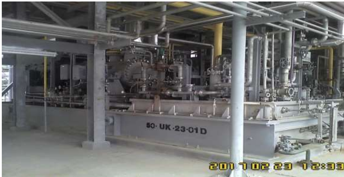
Figure II.13: Les Re-compresseurs.
