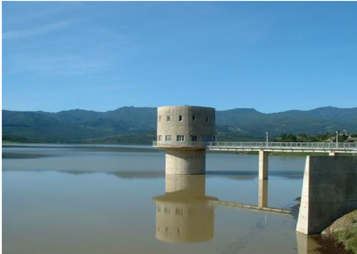
Figure 28: Barrage Beni Zid (74)
