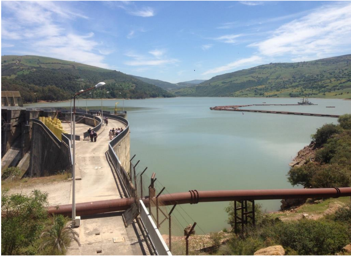
Figure 26: photo barrage de zerdas (73)
