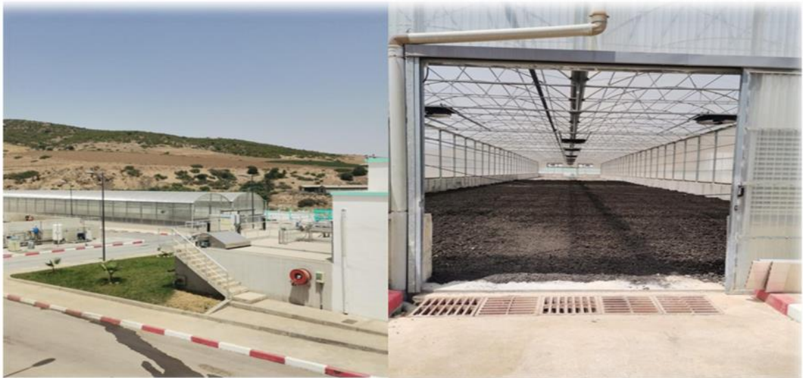
Figure III.15 : installation de séchage.
