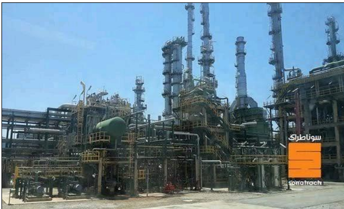
Figure II.1 : la raffinerie de Skikda RA1K
