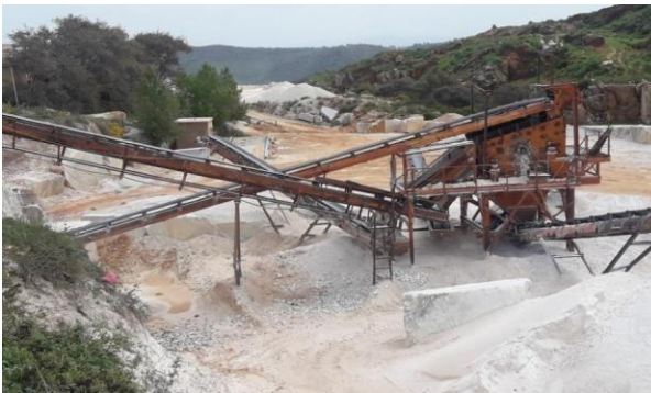
Figure 67. Station de concassage.
