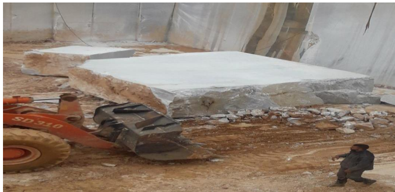
Figure 69. Chute des blocks extraits.
