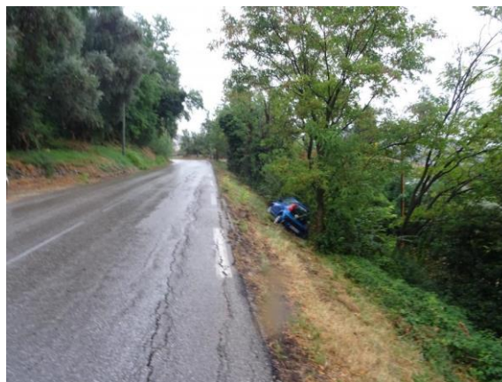
Figure II.3. Affaissement [29].
