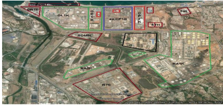
Figure II.1: Satellite view of the SKIKDA industrial zone.
