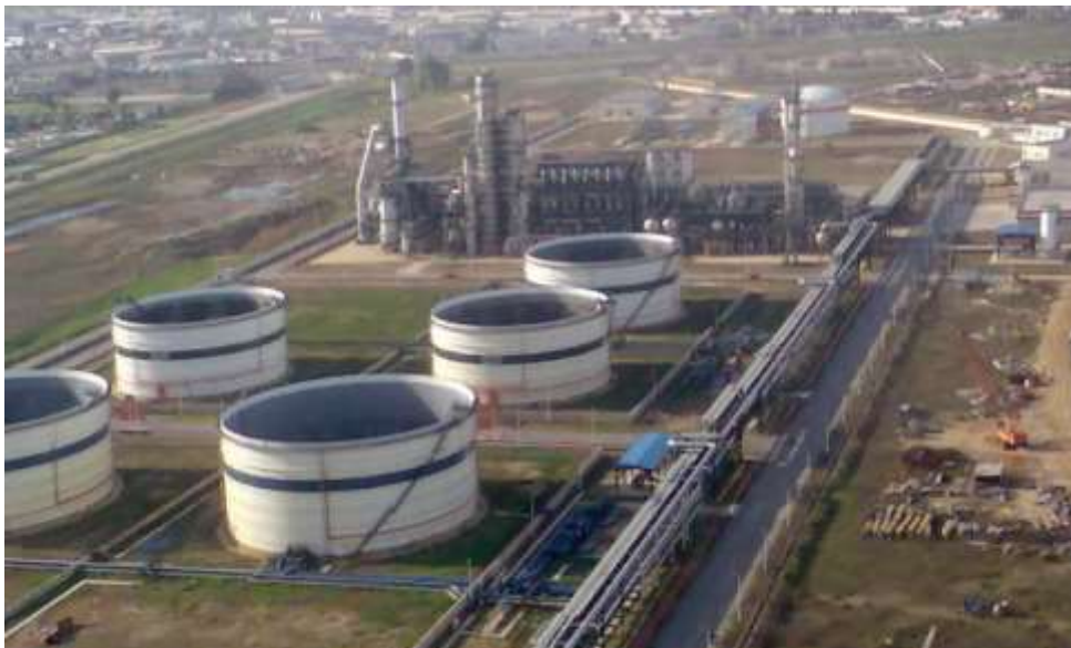
Figure III.1 : Station du Topping.
