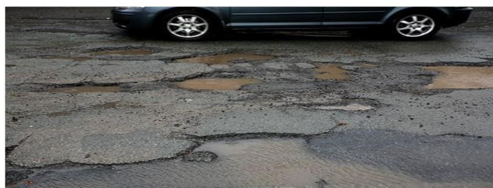
Figure 13 : Arrachement
