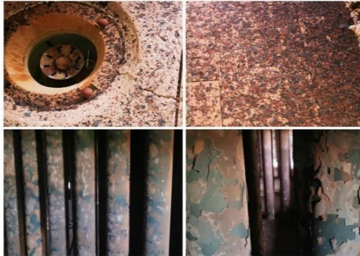
Figure 3.14: the inspected radiant tubes.
