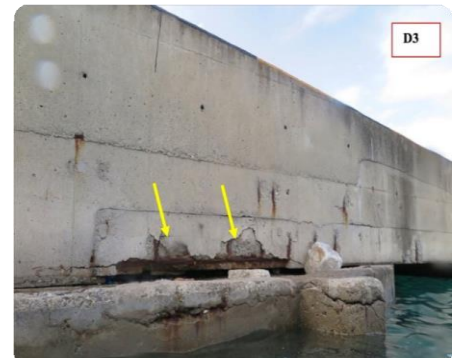
Figure II.14. Ecaillage.
