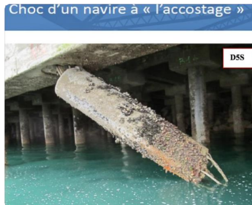
Figure II.7. Fracture.
