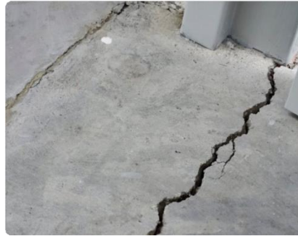
Figure II.9. Fissuration.
