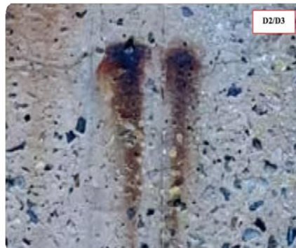
Figure II.11. Carbonatation.
