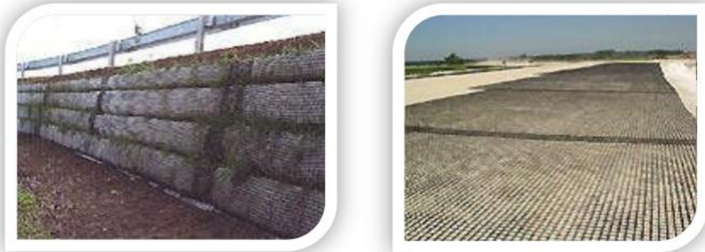
Figure 8: Renforcement de sol
